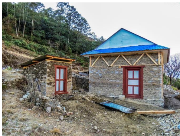
Earthquake-proof house and toilet built in January 2019
