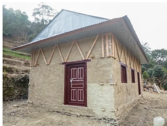
Earthquake-resistant house built in December 2020
