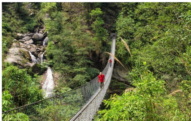
The metal bridge built in 2009
