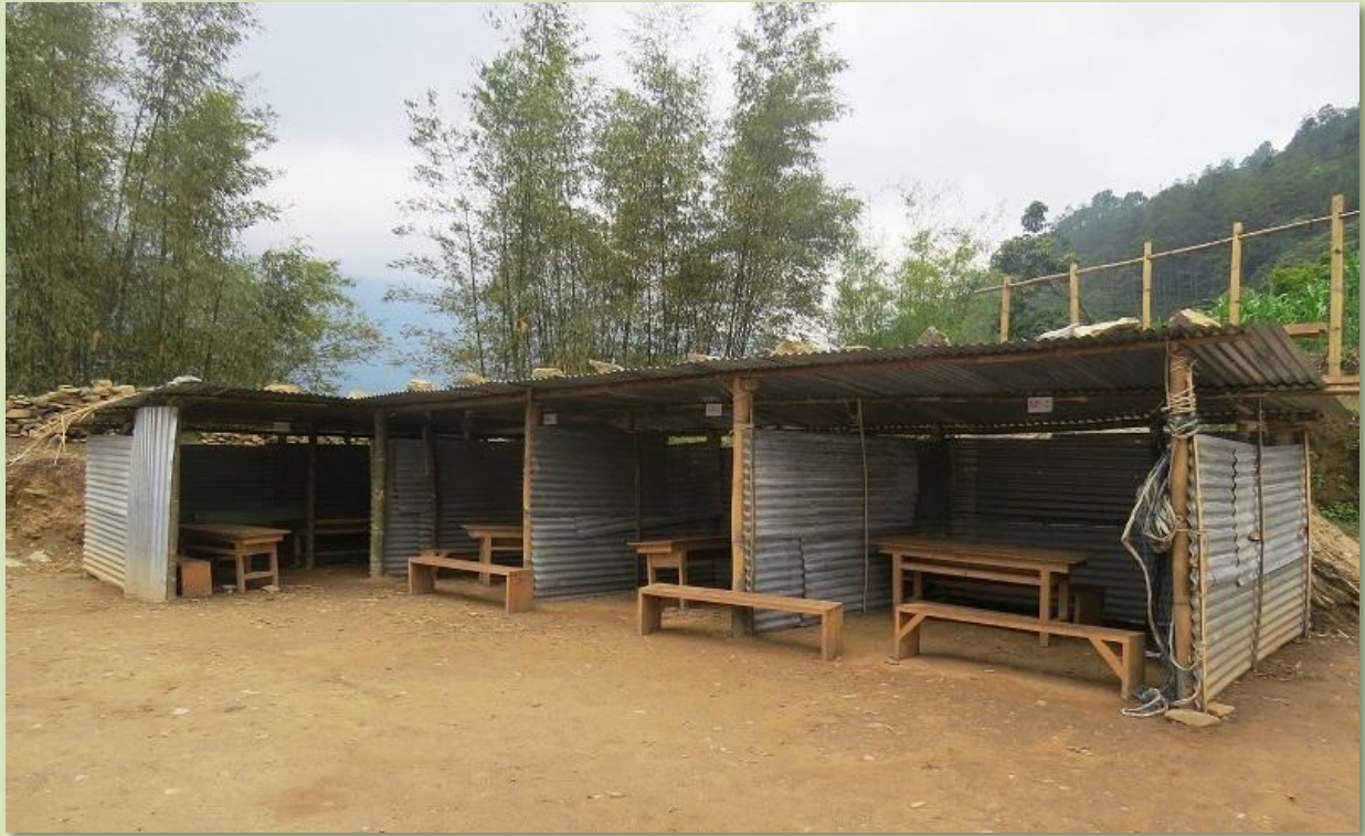
A temporary classroom at Lop pre-primary School
